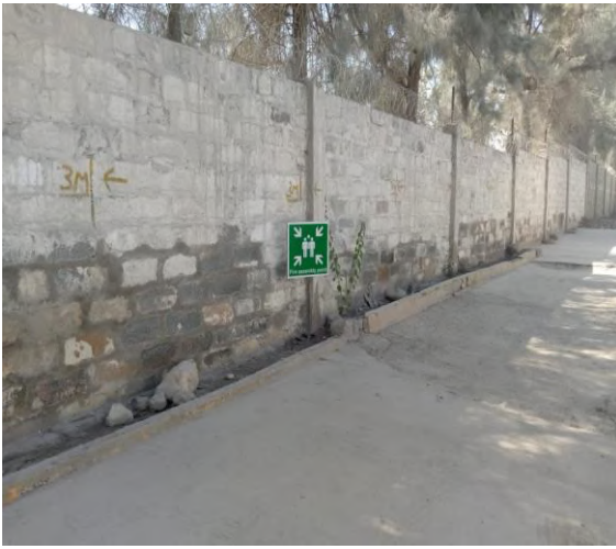
Perimeter Wall Within the Site
