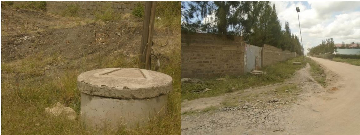
Plate 16: Existing MAVWASCO sewer line manholes in the area
