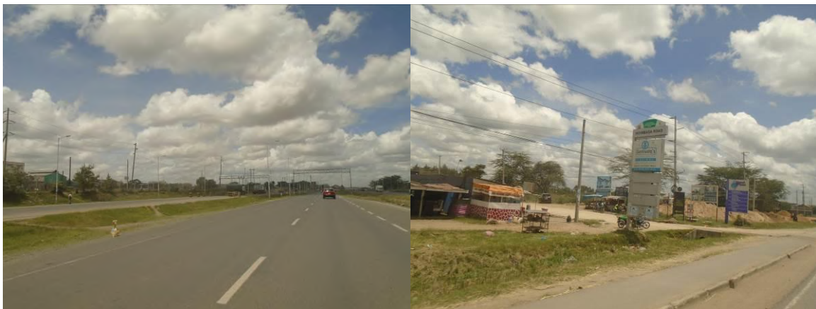
Plate 11: Section of Mombasa- Nairobi Highway and junction of Muthama Access Road
