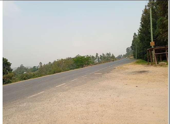
Plate 4: Main tarmac Eshikinji- Esumeiya access road to the site
