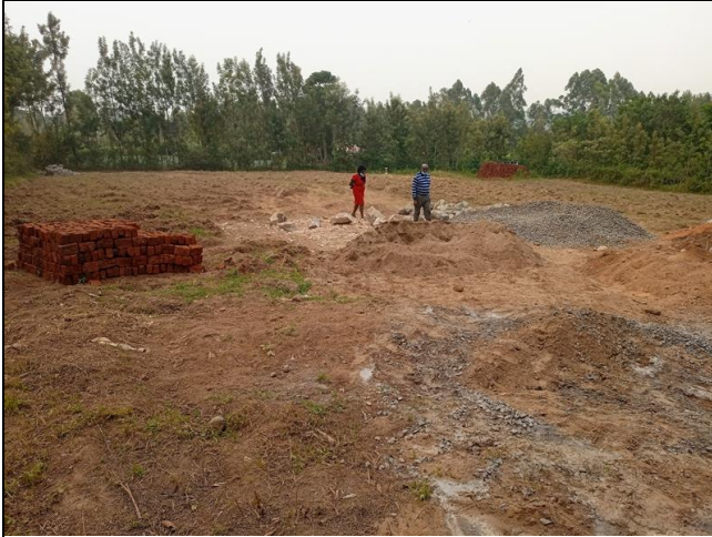
Plate 3: Proposed project site and some few construction materials on site
