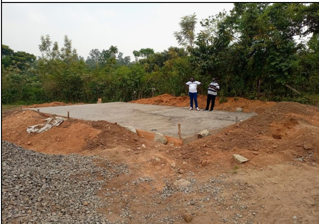
Plate 5: Site house currently under construction.
