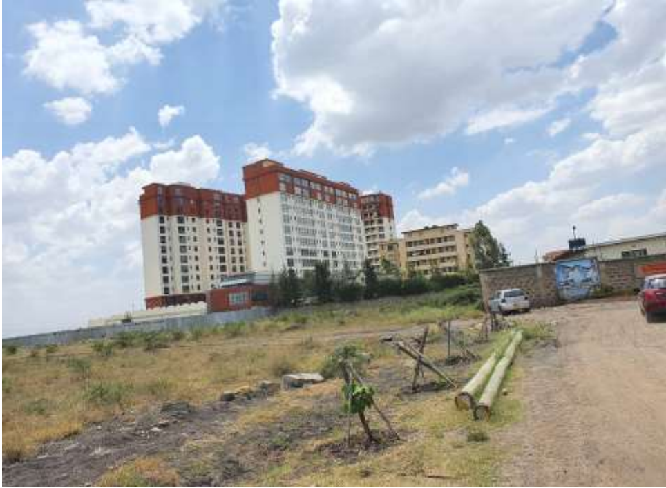
Proposed construction site and the adjacent developments on the western edge
