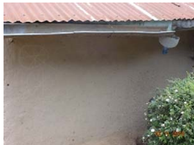
Figure 14: Roof Rain Water Harvesting
