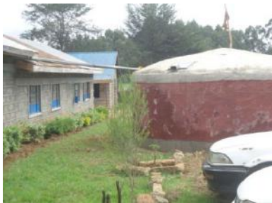
Figure 14: Roof Rain Water Harvesting
