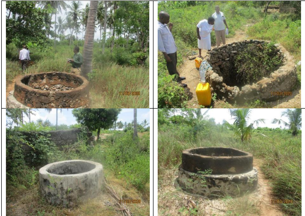
Plate 6: Identification of boreholes
