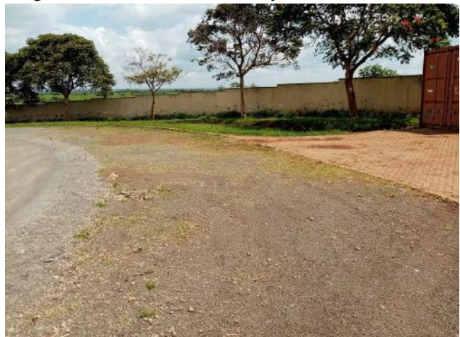
Section of perimeter wall that goes all round the site
