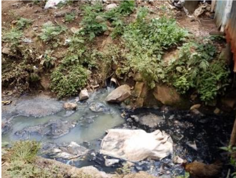
Plate 4: Raw sewage released into storm water drainage
