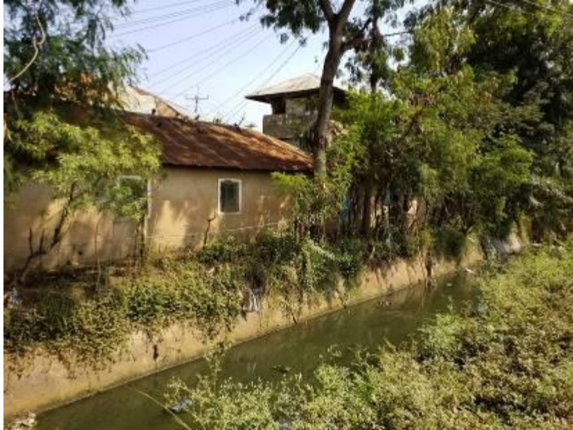
Plate 5: Structures along Auji line likely to be affected
