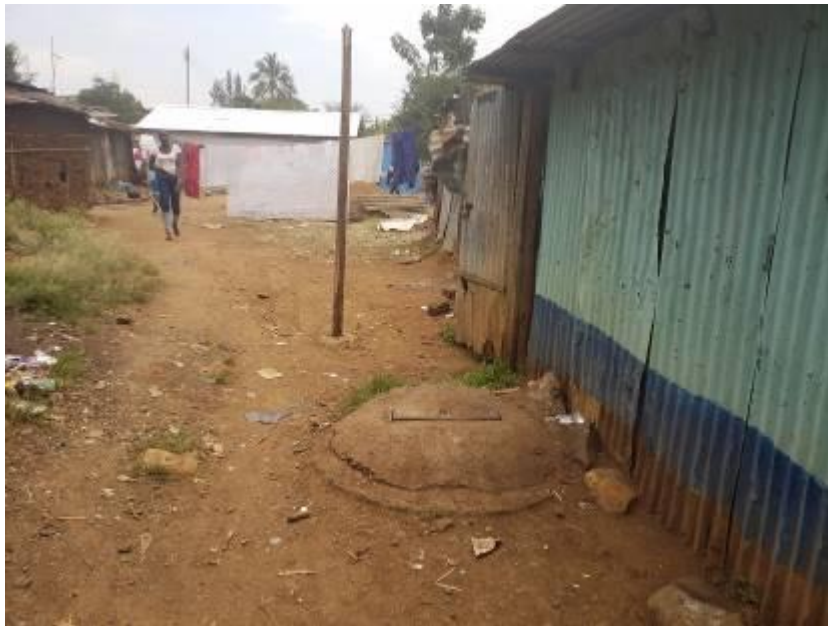
Plate 7: Structure located along Kenya Brewery sewer line
