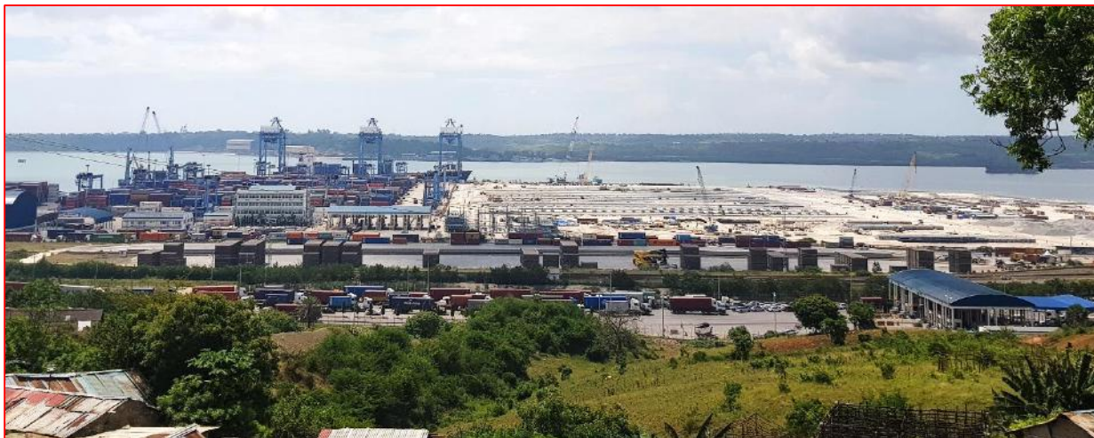
Figure 13: A section of Kenya Ports Authority (Container Terminal 2 and the ongoing construction of Mombasa Port Development Plan Phase 2) neighboring the project site (Source: Site visit, November 2020).
