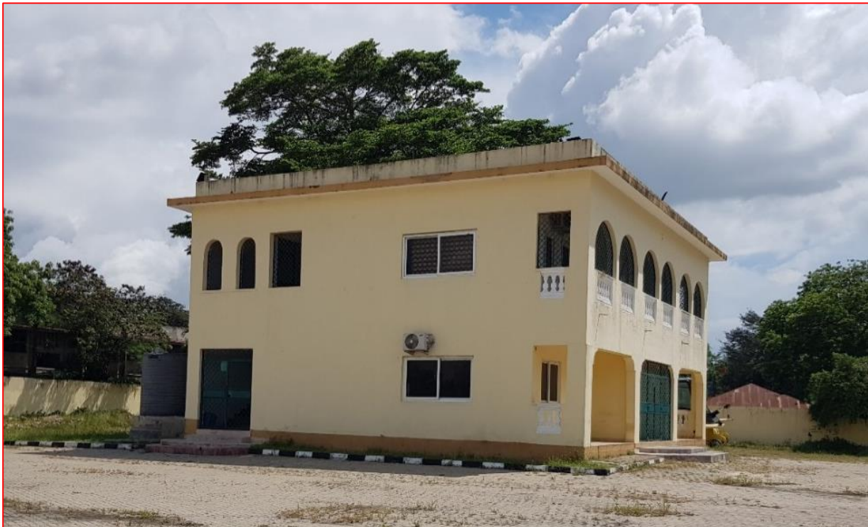
Figure 5: The existing one storey administration block (Source: Site visit, November 2020).
