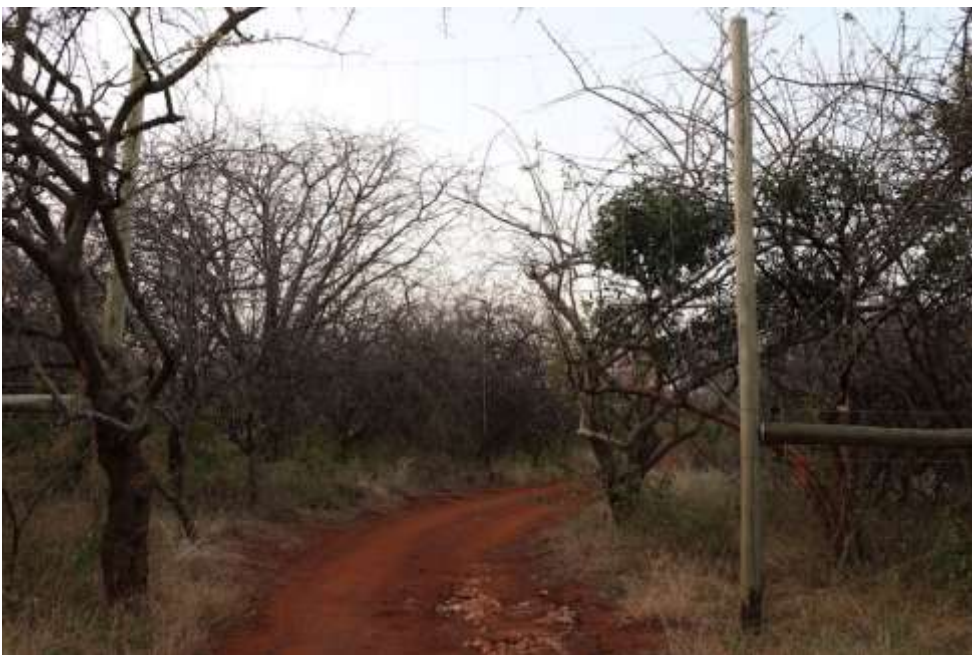
Fig 13. Photo shows a road pass through the Elephant Exclusion Zone style fence, with 2 x 20-foot posts on either side of the road holding up the electric wires with “drop down wires” to allow vehicles to pass underneath.
