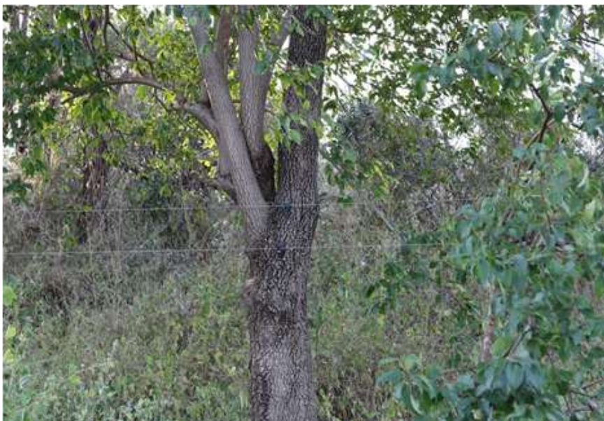
Fig 11. Photo shows 2 wire strands attached to a live tree, using W-insulators, where the tree acts as the support instead of a fence post.
