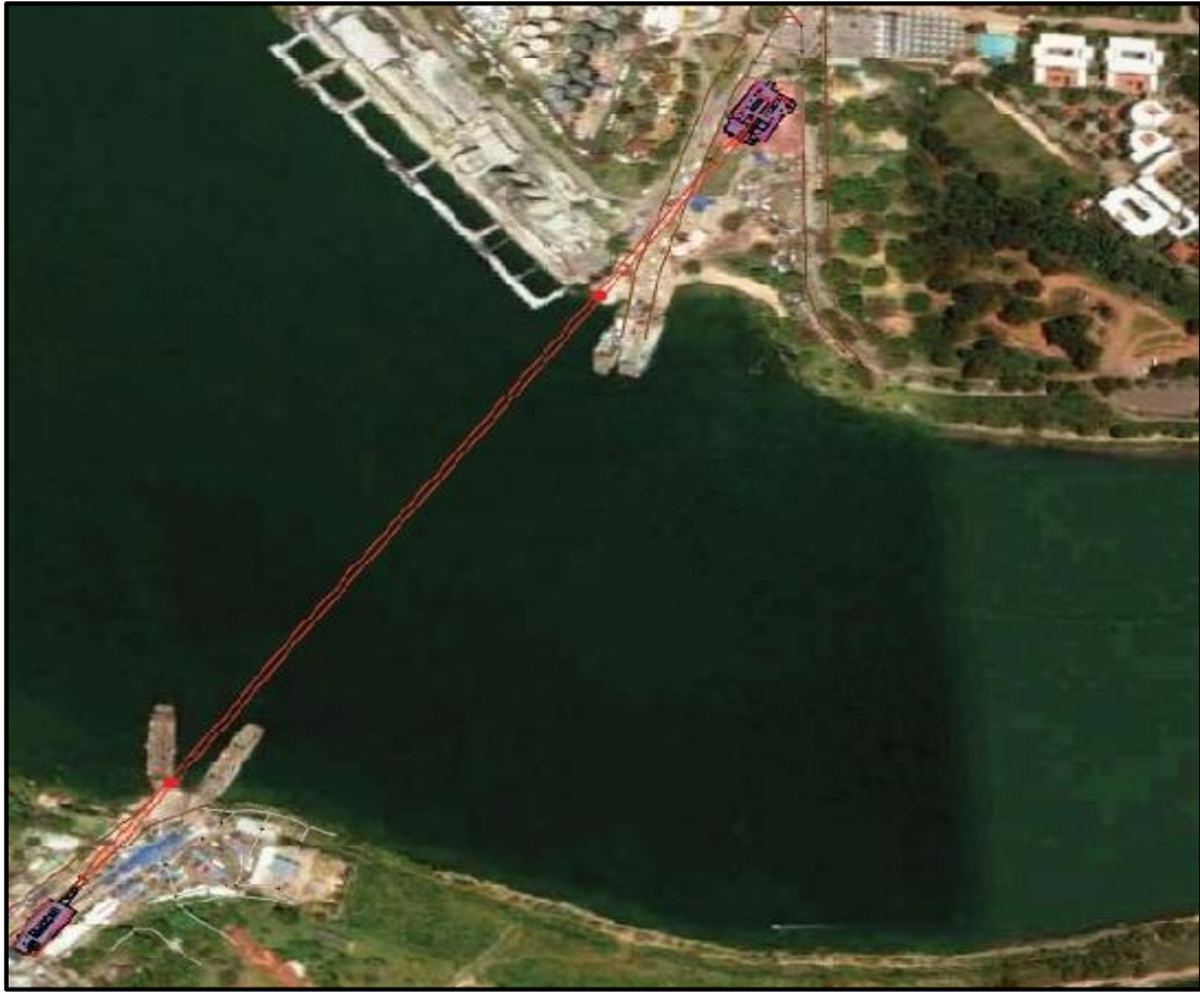
Figure 6. 13: Alignment across the channel
