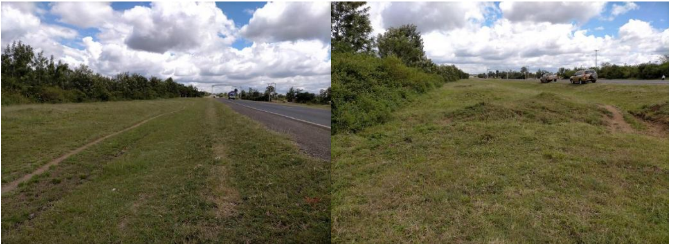
PROJECT ACCESS SITE ACCESS ROAD- THIKA – GARISSA HIGHWAY
