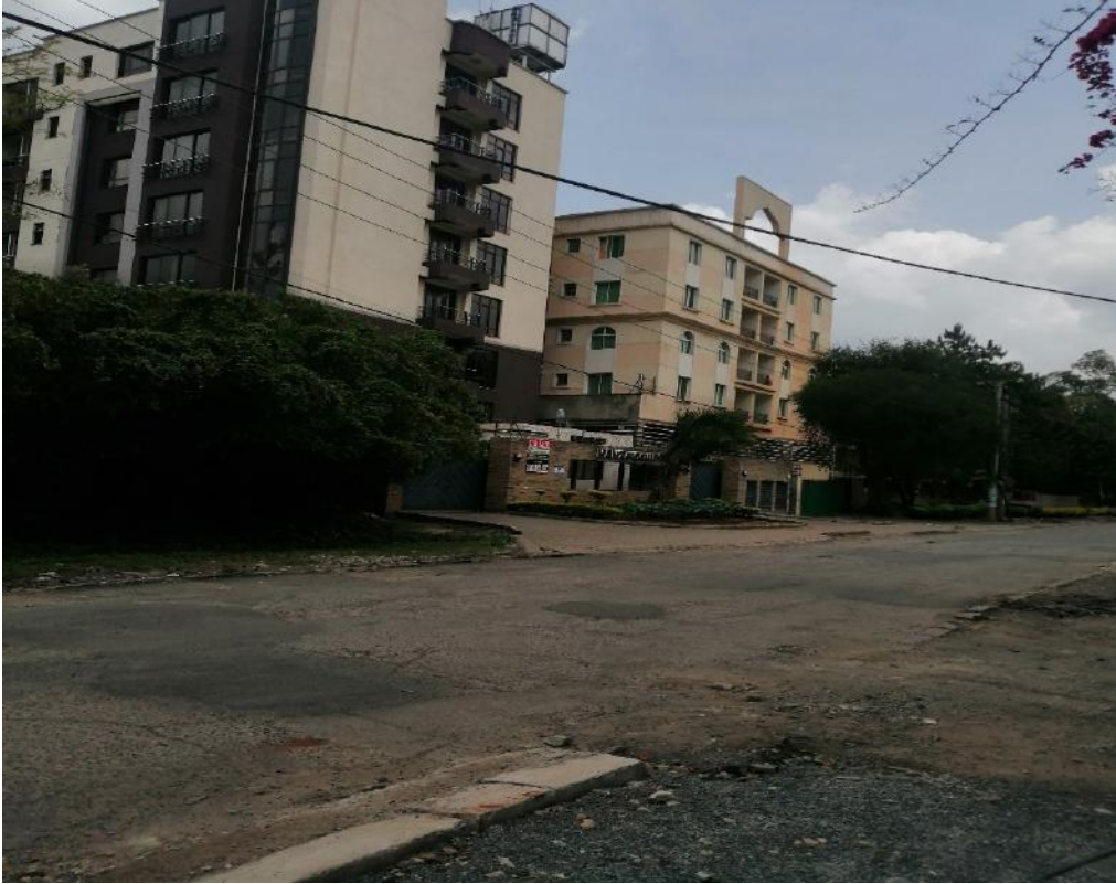
Figure 2 Neighbouring residential properties similar to the proposed project
