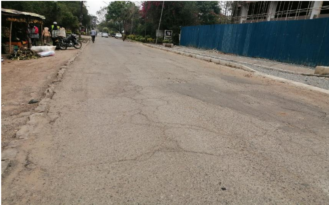
Figure 4 Access road to the site (Kirichwa Road)
