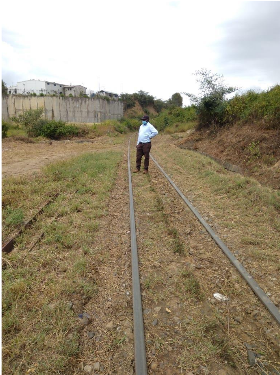
Photo 7: A Railway Line passing next to the Proposed LPG Plant Site at Kibarani, Kipevu area
