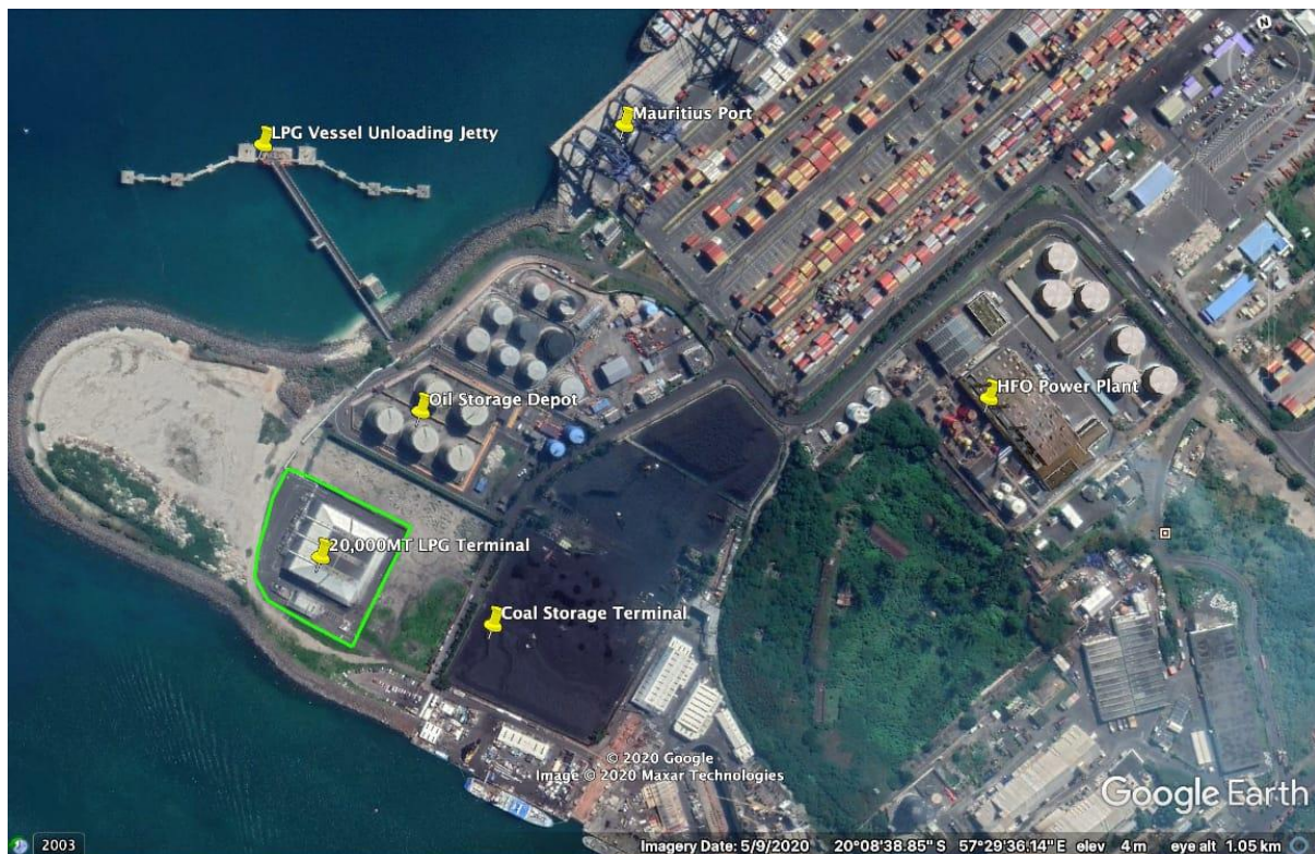
Fig 1: Mapping giving the location and neighbourhood of the 20,000 metric tons LPG storage depot in Mauritius
