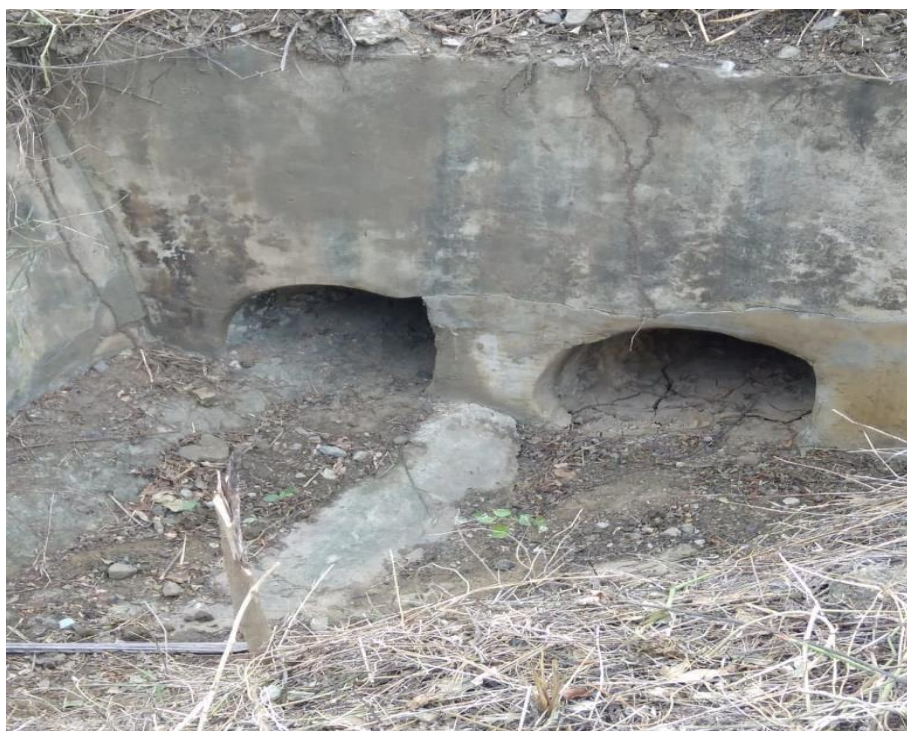
Photo 7: The Storm water drainage on a section of the proposed site
