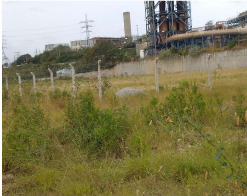
Photo 8: The Existing Kengen, Kipevu 1 Plant neighboring the proposed site
