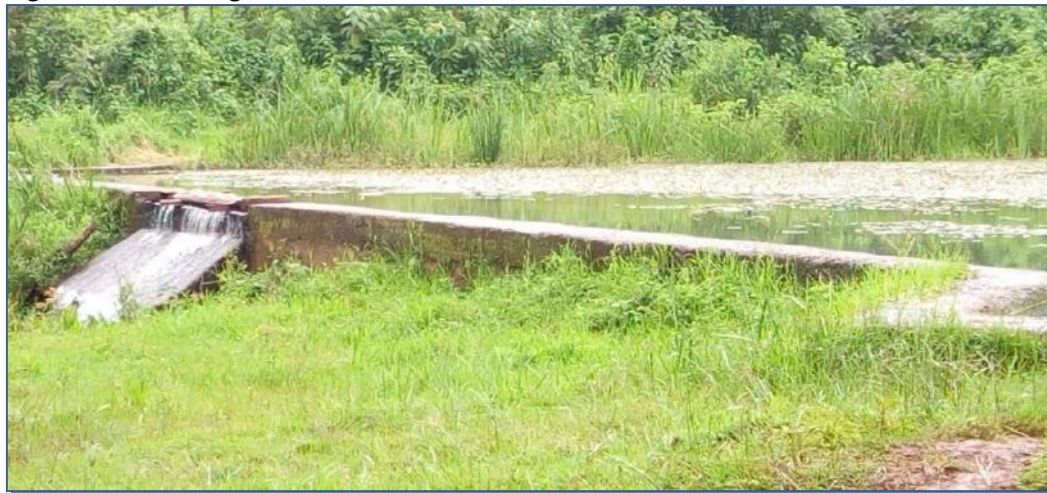
Figure 2-1: Existing Taito dam
