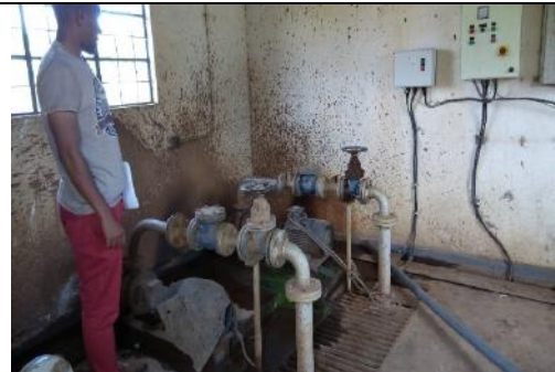
Photo-plate 1-2: Raw Water Pumps
