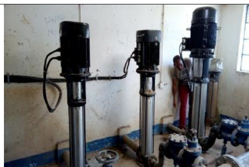
Photo-plate 1-4: Configuration of the existing high lift vertical mounted pumps
