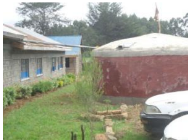
Figure 14: Roof Rain Water Harvesting
