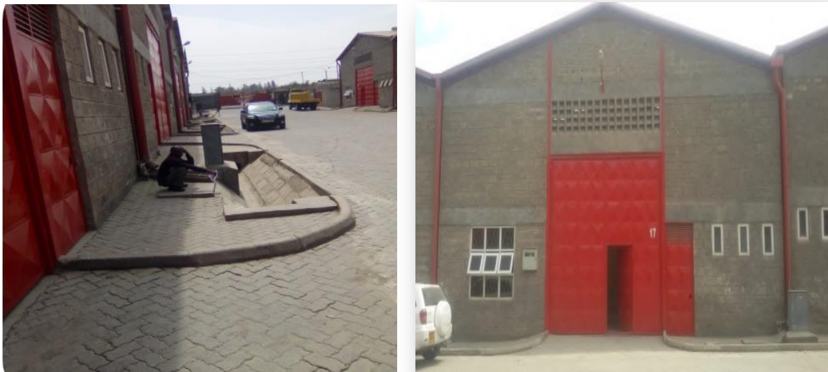
Figure 5: Photo showing the Scarlet Business Park
