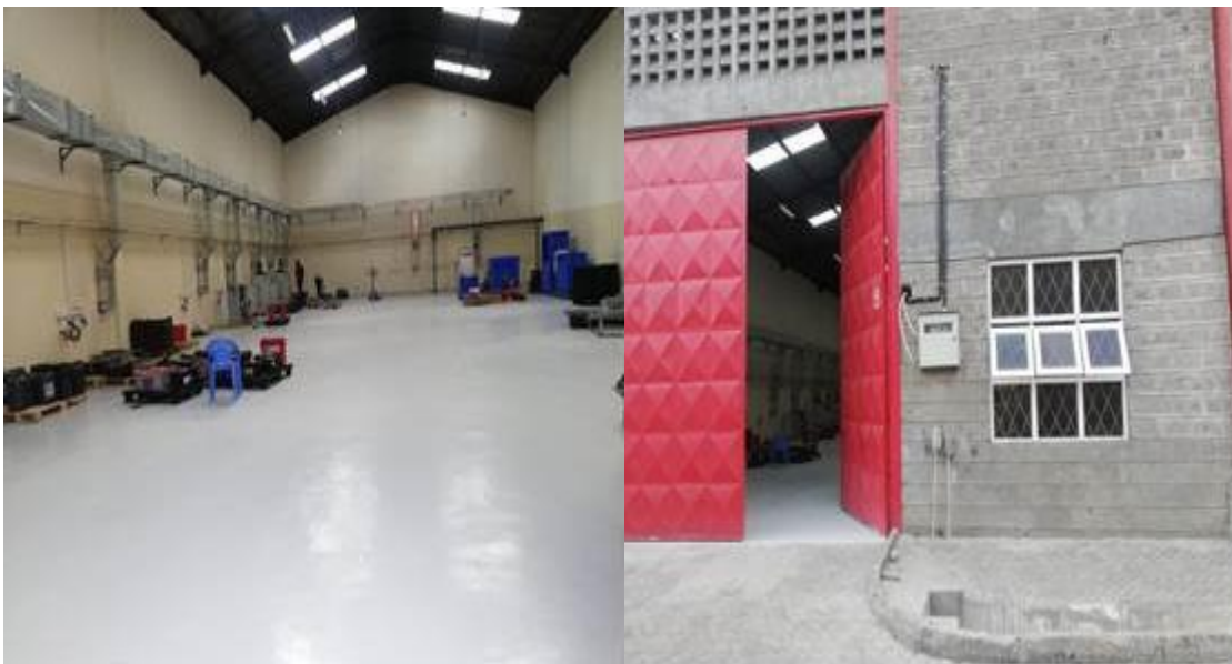
Part of the Rented Warehouse where the proposed Plant will be Located
