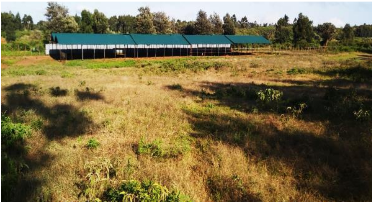
Figure 4: Some of the large roof surfaces to be utilized for rain water harvesting
