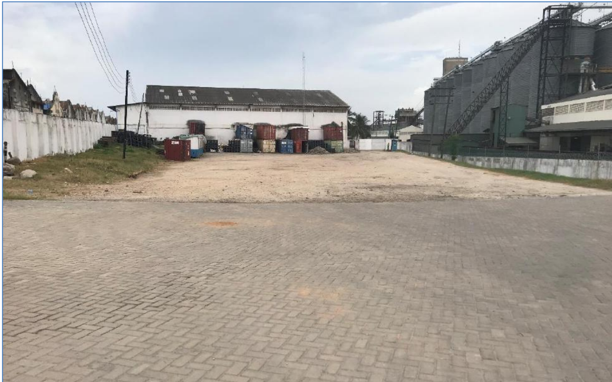
Figure 7: A section of the proposed project site (Source: site visit, March 2020).
