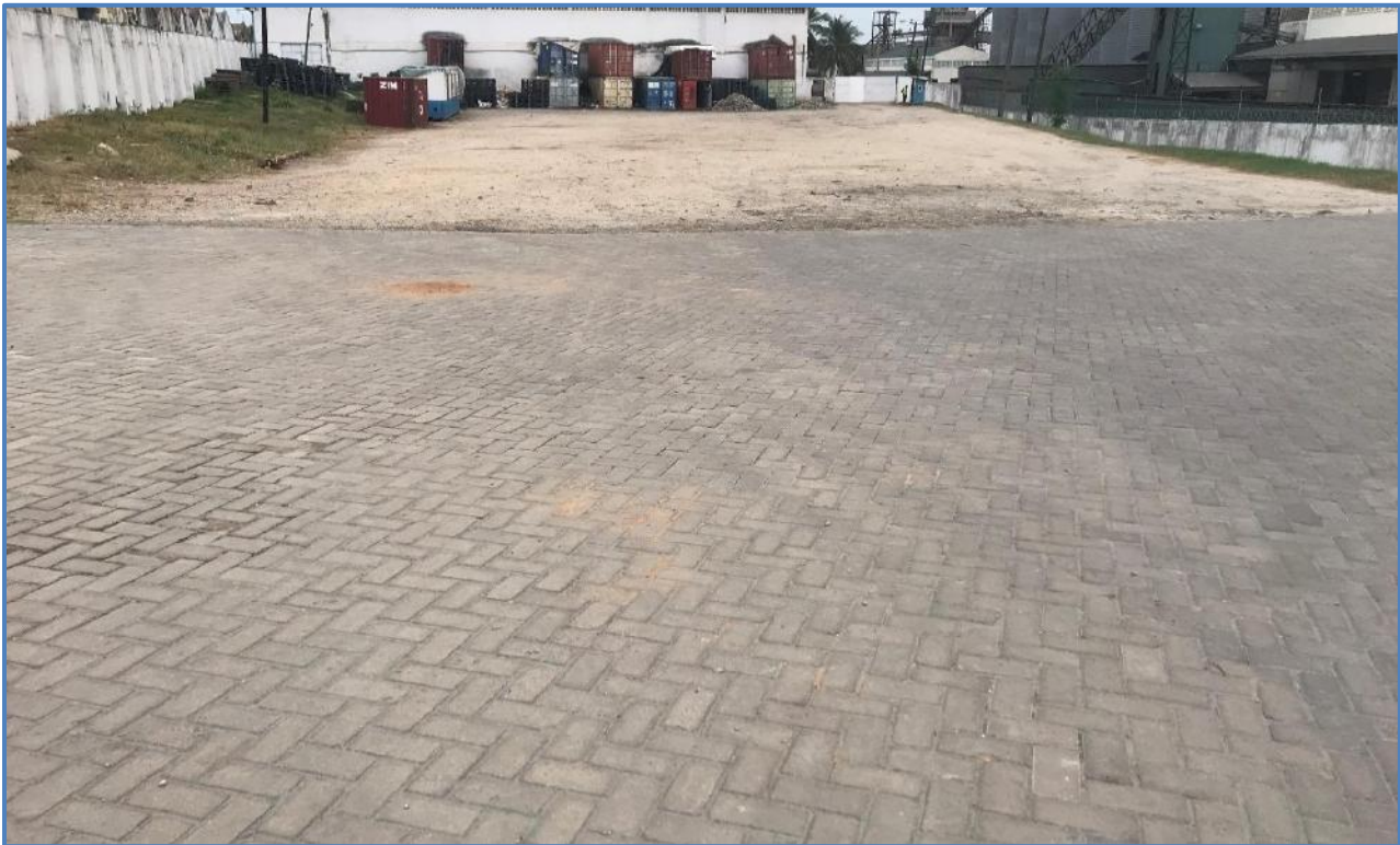
Figure 3: A section of the proposed project site (Source: Site visit, March 2020).
