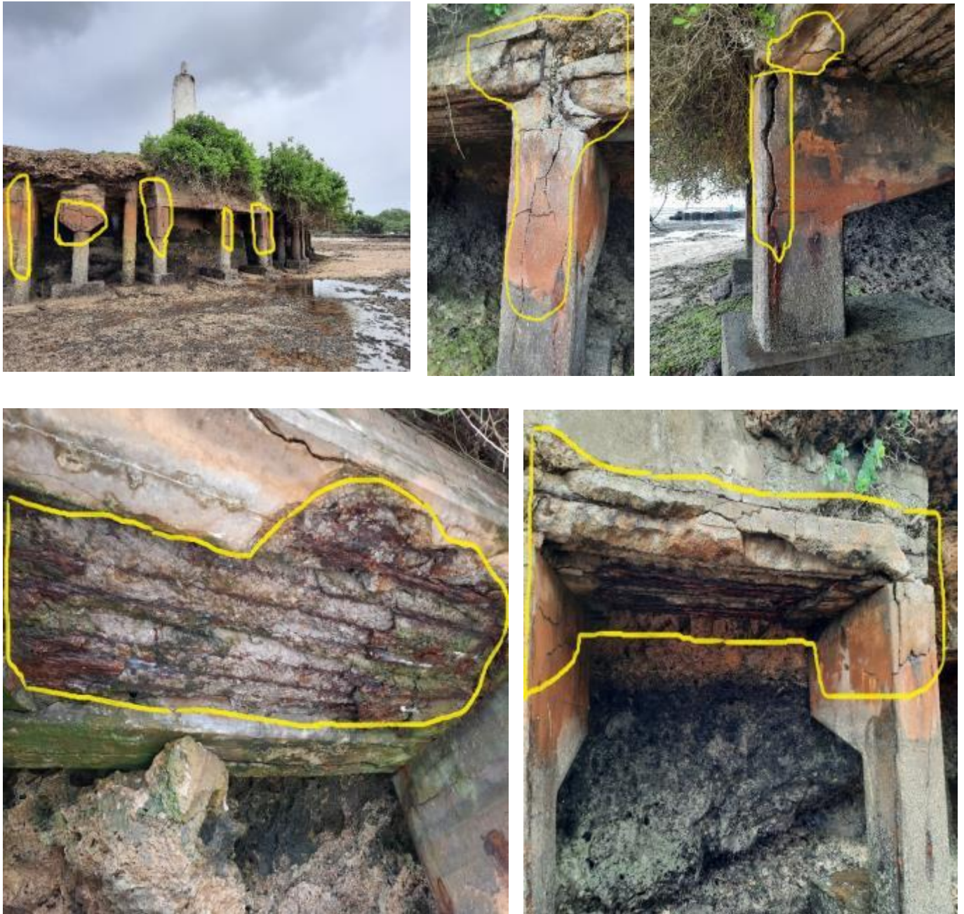
Figure 6: Photos of Extensive damage to the pillars supporting the Base Rock of Vasco Da Gama pillar
