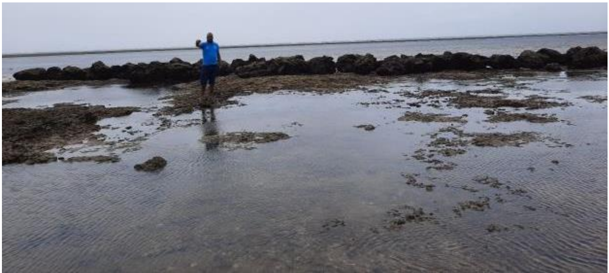
Figure 24: A collection of rock boulders placed to Prevent Erosion of the Vasco Da Gama pillar
