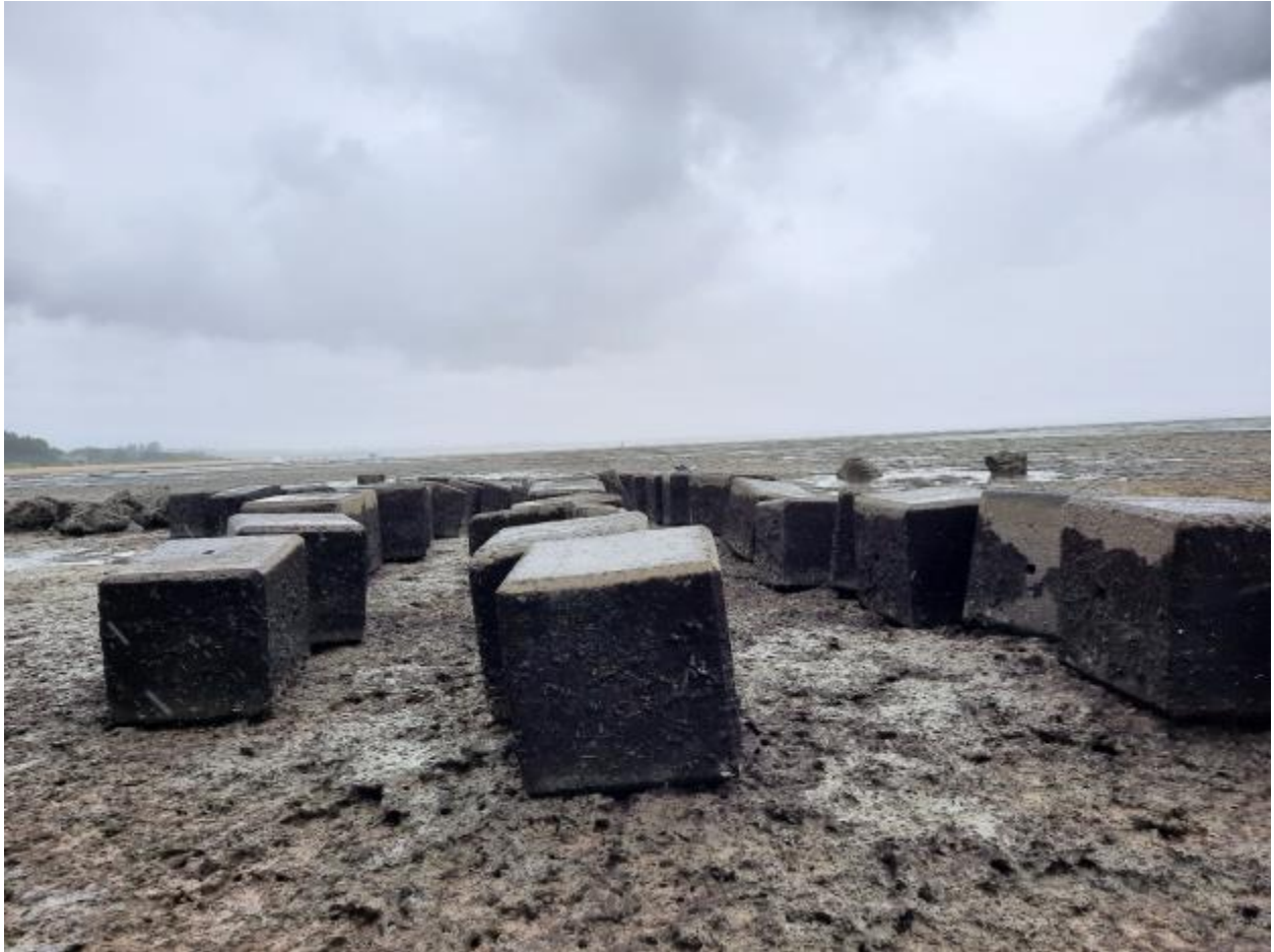
Figure 23: Collection of Concrete Blocks Placed at the northern edge of Vasco Da Gama pillar as Wave Energy Breakers
