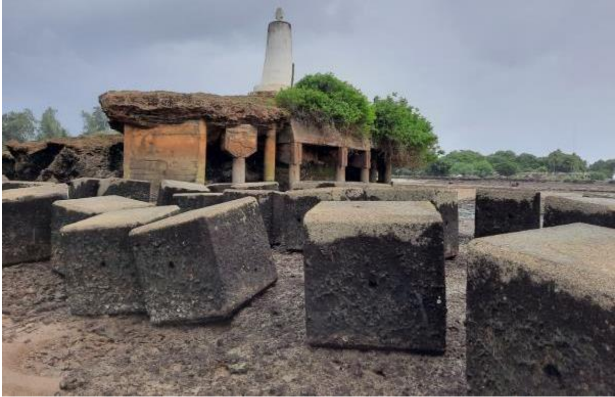
Figure 21: A view of previous efforts to support the reef terrace using reinforced concrete pillars and reduce the velocity of waves using concrete boulders.
