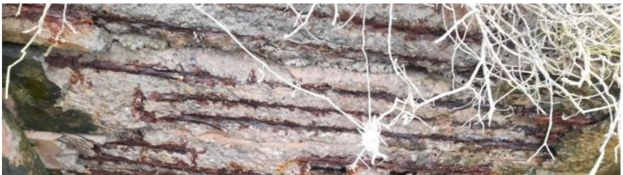
Figure 22: Eroded Sections of the support pillars of Vasco Da Gama promontory
