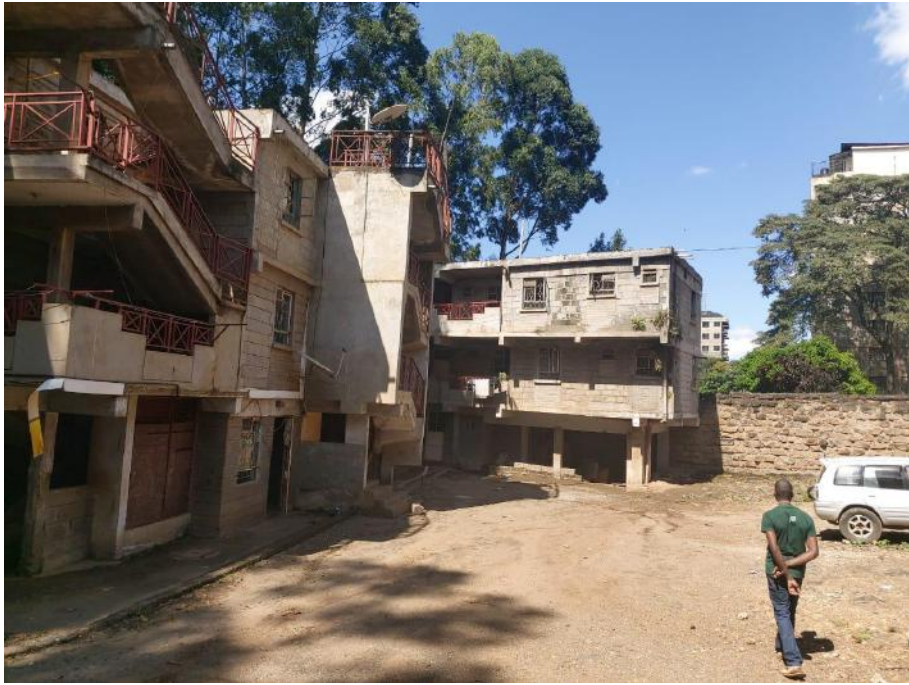
Figure 4: Showing existing structures on the plot
