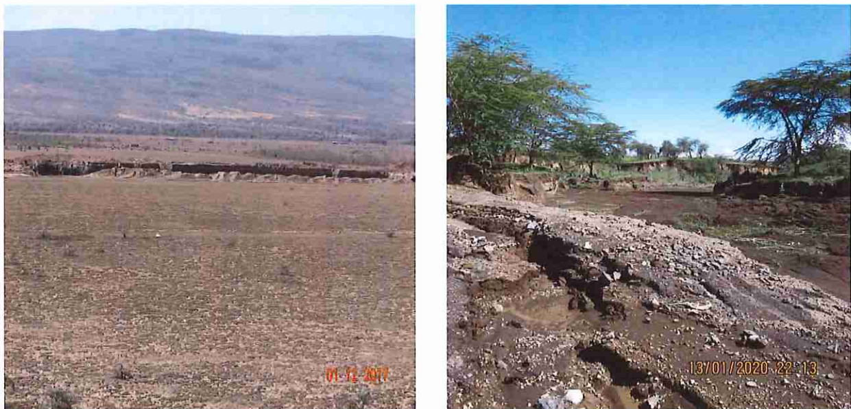
Typical Surface Drainage Channels. Note the Erosion Features due to Non-Cohesive Soils
