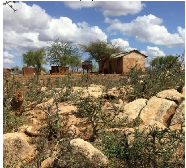
Plate 1-4: Existing permanent house structures on the proposed site
