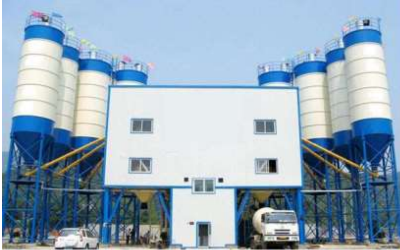
caption 2: Example of Concrete mixing station
