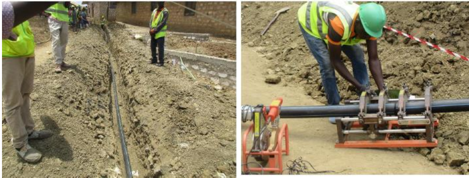
Figure 4-3. Typical construction and laying of pipeline
