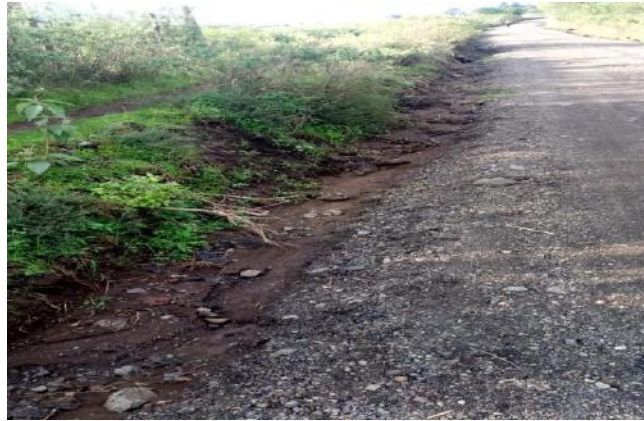
Plate 6.5: Typical road section leading to the project site
