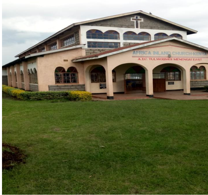
Plate 6.9: AIC Tulwobmoi Church shares the fence perimeter with the project site.
