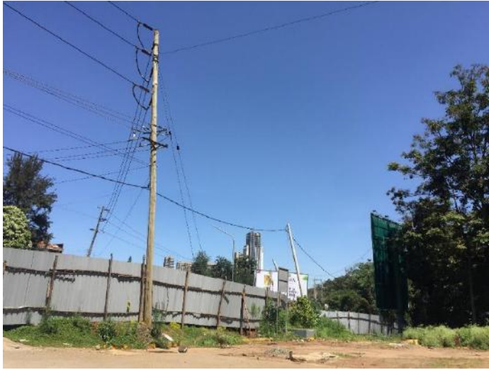
Photo 14: Electricity supply right at the site
