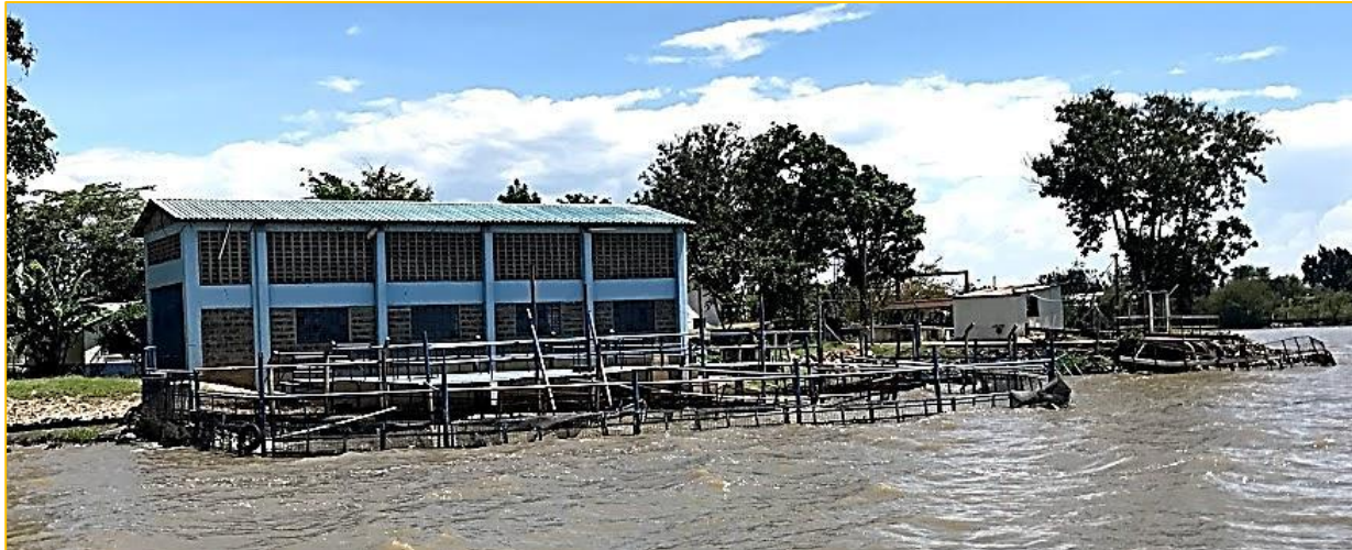
Figure 39. Municipal water intake point at Dunga beach on the shores of Lake Victoria (Source: Site visit, November 2019).
