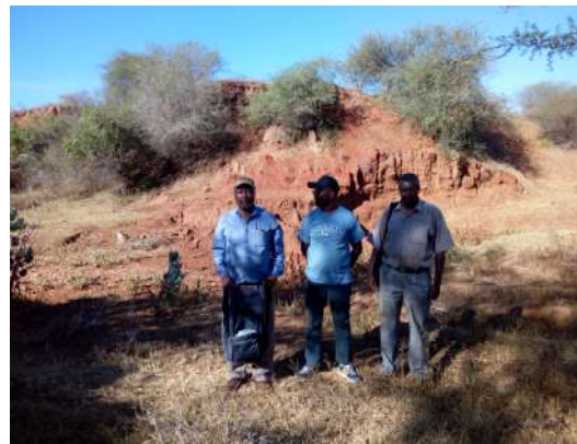
The Social Services Coordinator-Mr. Mbui, ESIA Lead Expert- Mr. Quentin and Irrigation Engineer Mr. Musyimi standing before the previous destroyed dam wall
