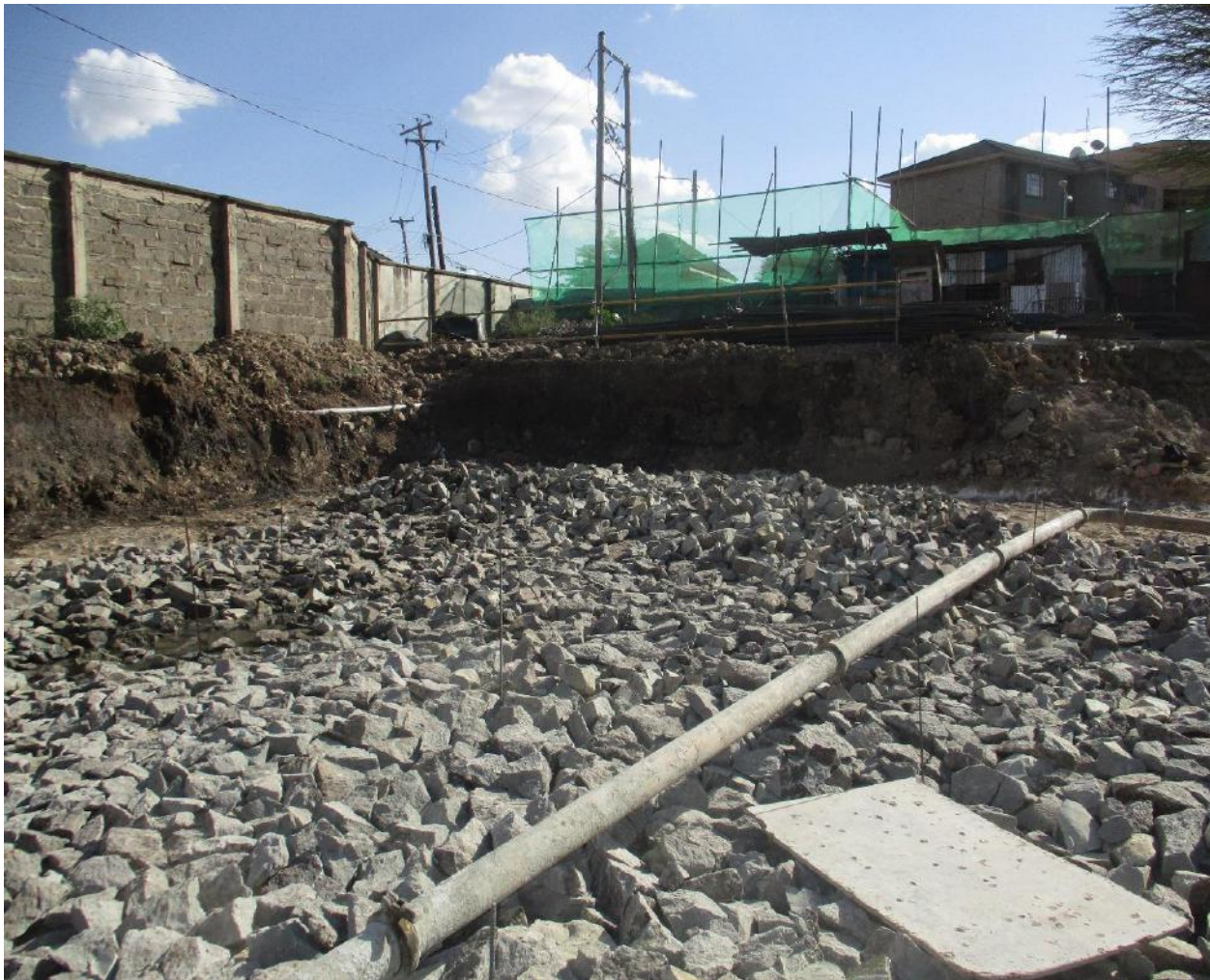
Figure 1: Photo Showing The Proposed Development Project Site
