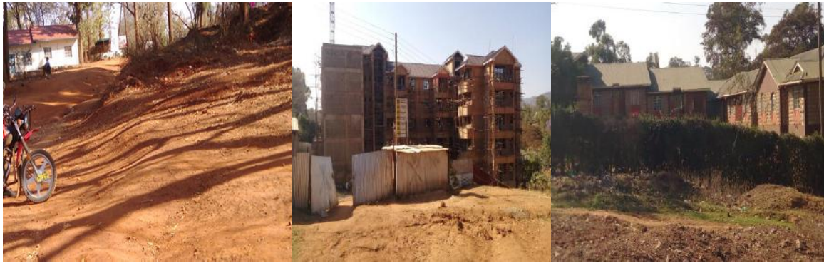
Figure 7 Neighbours to the site - NIS office, private development and police lines
