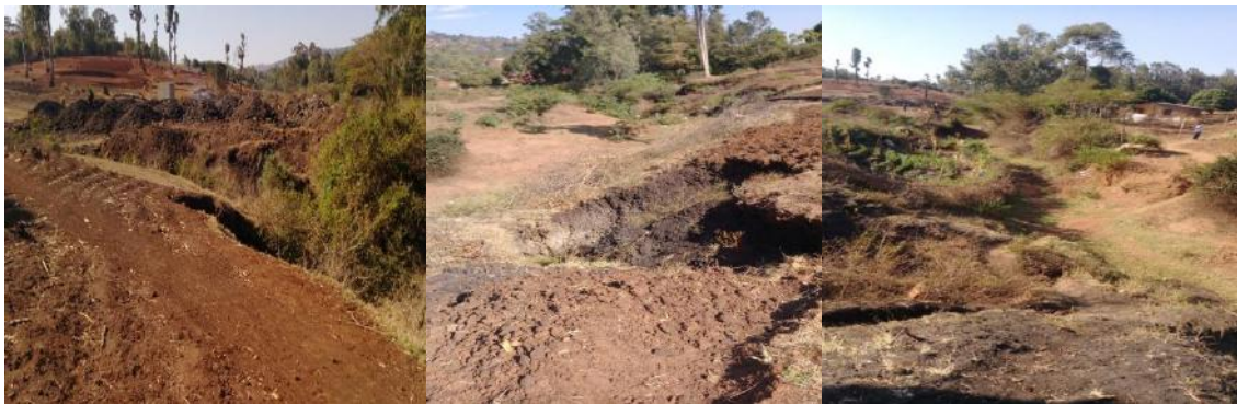
Figure 8 River line = effects of soil erosion damage the riparian
