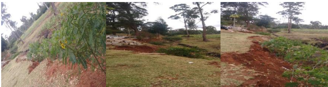
Figure 9 Stream abutting the site = effects of storm water damage on riparian
