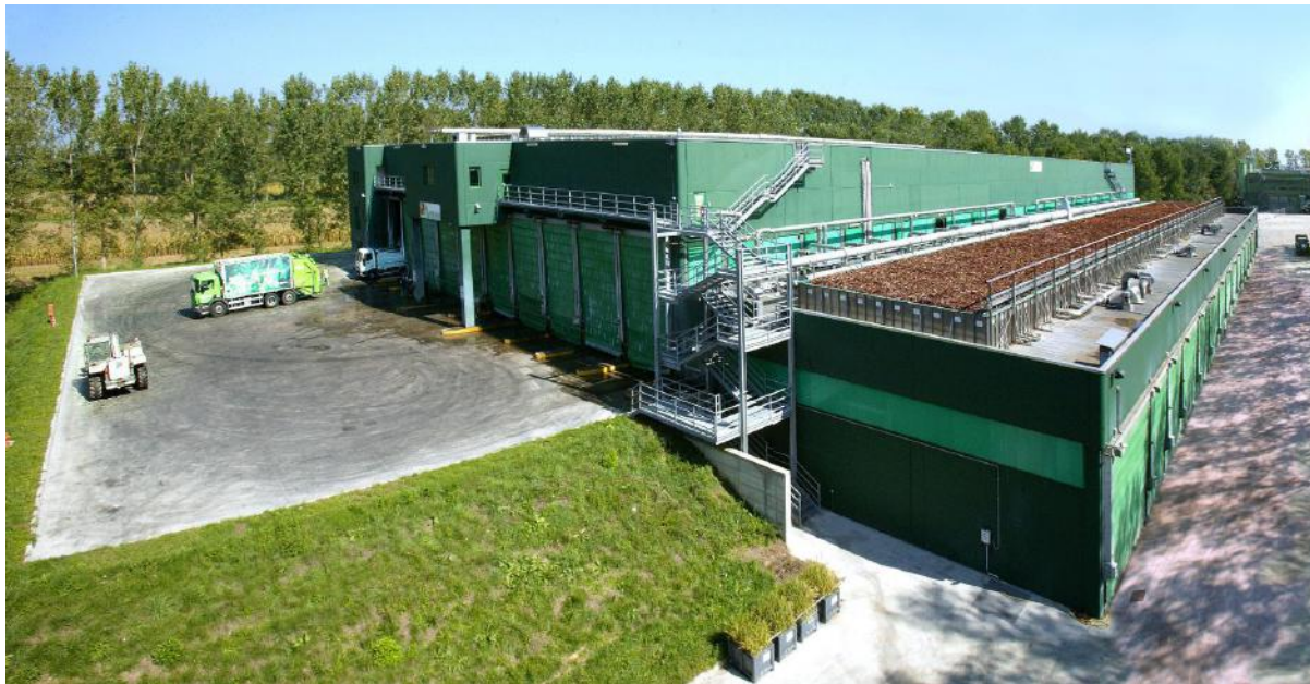
Plate 2 Bio-drying building and the coupled bio-filter on the roof
