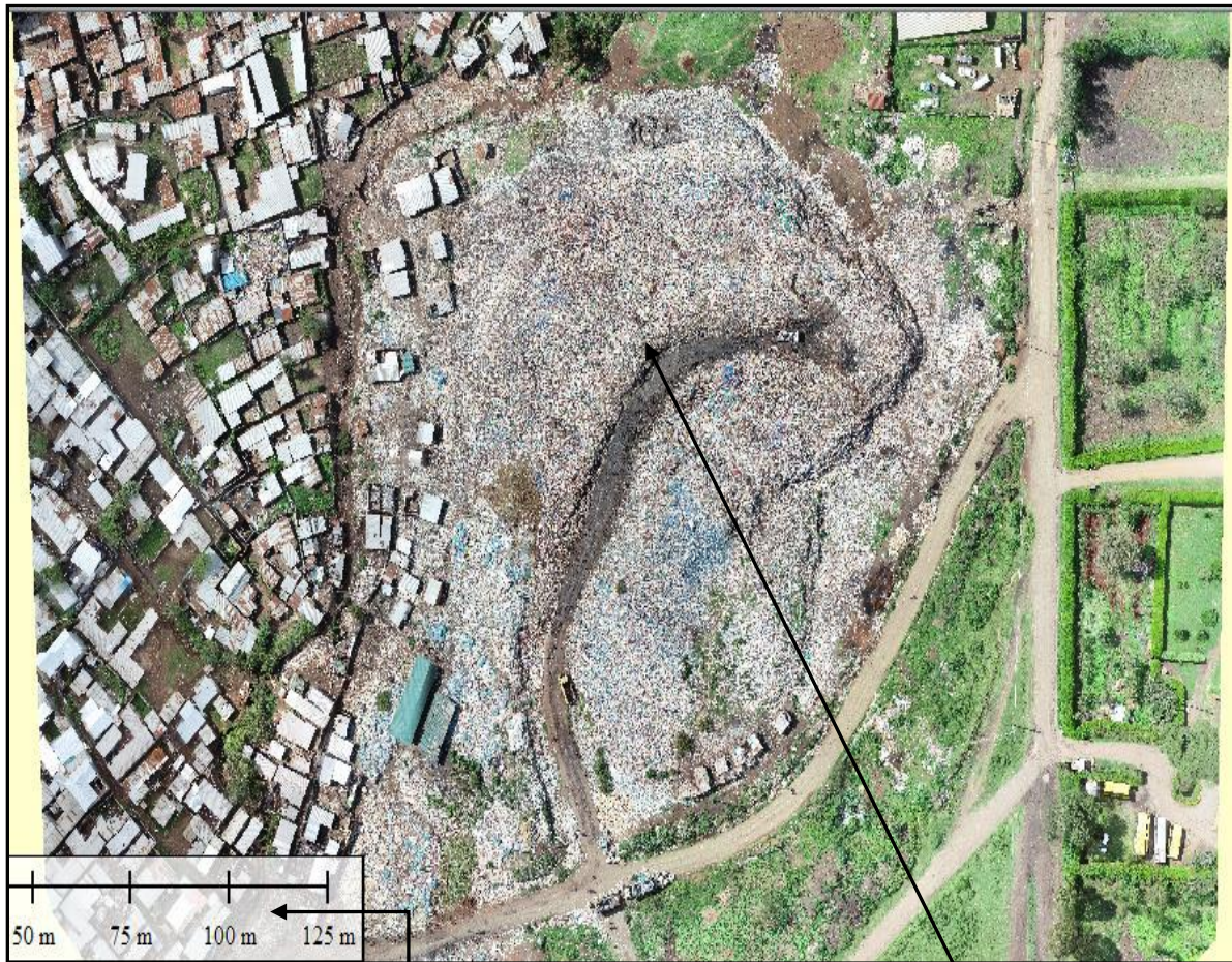
Figure 1: An Orth-mosaicked Image from UAV showing the dumpsite area Waste accumulated in the dumpsite Slum area Access road network
