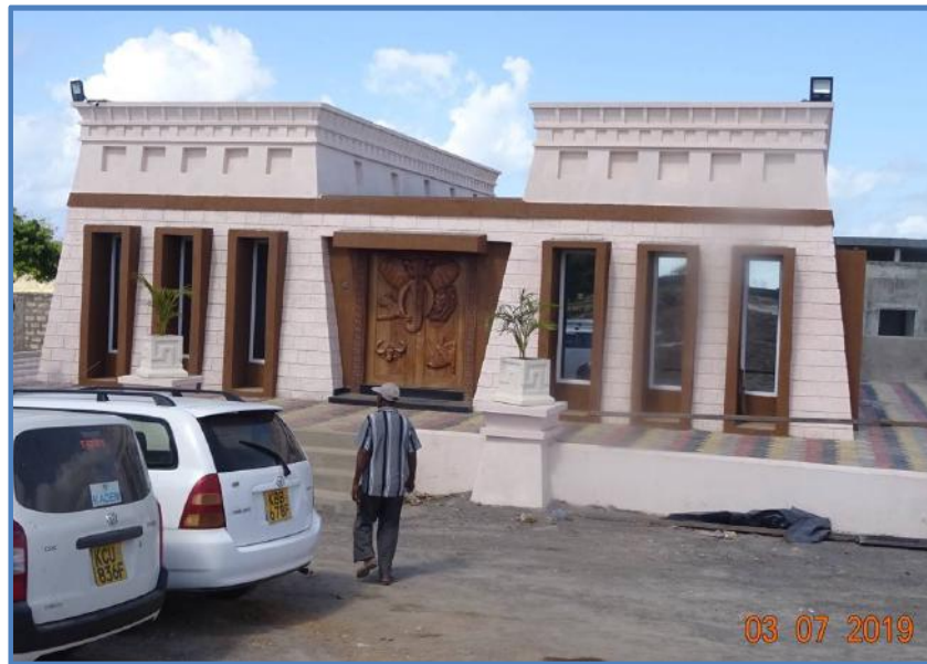
Figure 10 Completed show house/ site office at the project site
