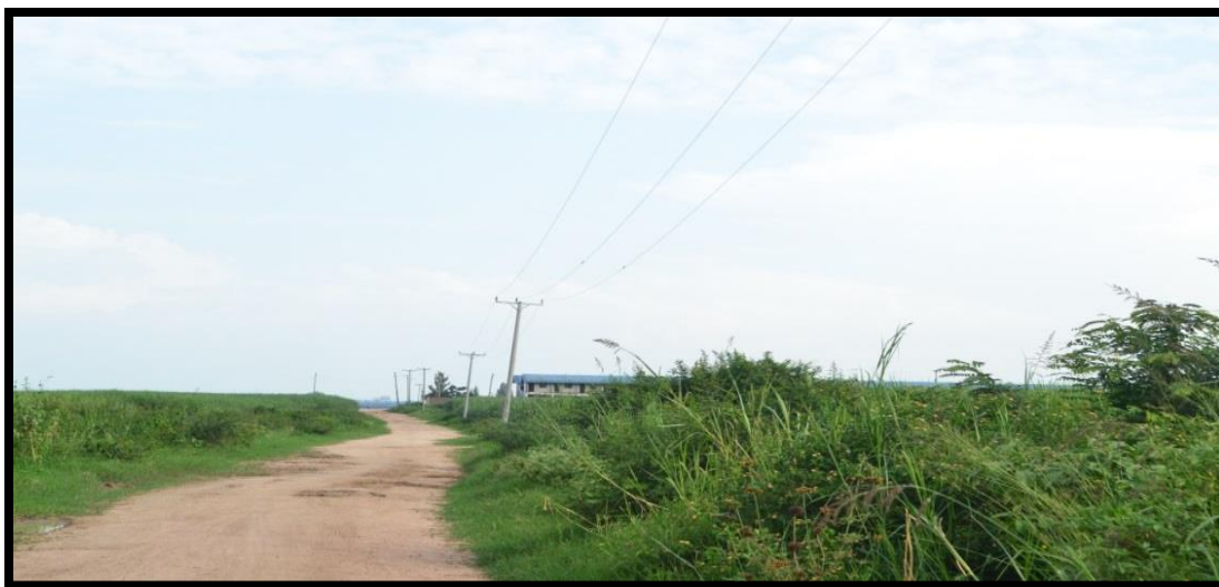
Plate 11: The Power lines from KSAIL Co-generation plant next to the proposed project site
