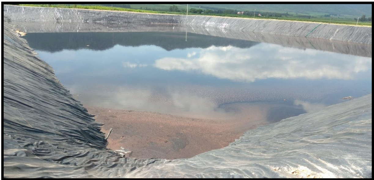
Plate 13: The DSW from the distillery storage lagoon next to the project site
