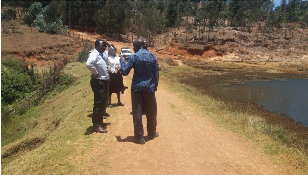
Figure 42 The leaking walls of the Exjacob dam
