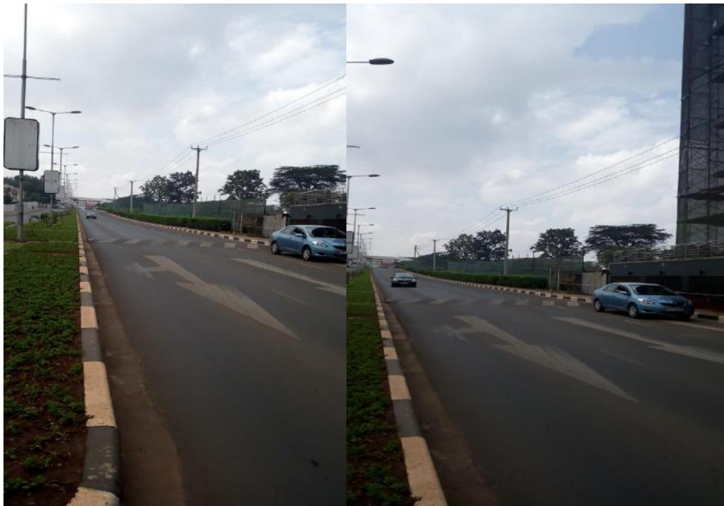
Boulevard road connecting the site, Ngumba Road and Garden City Mall
