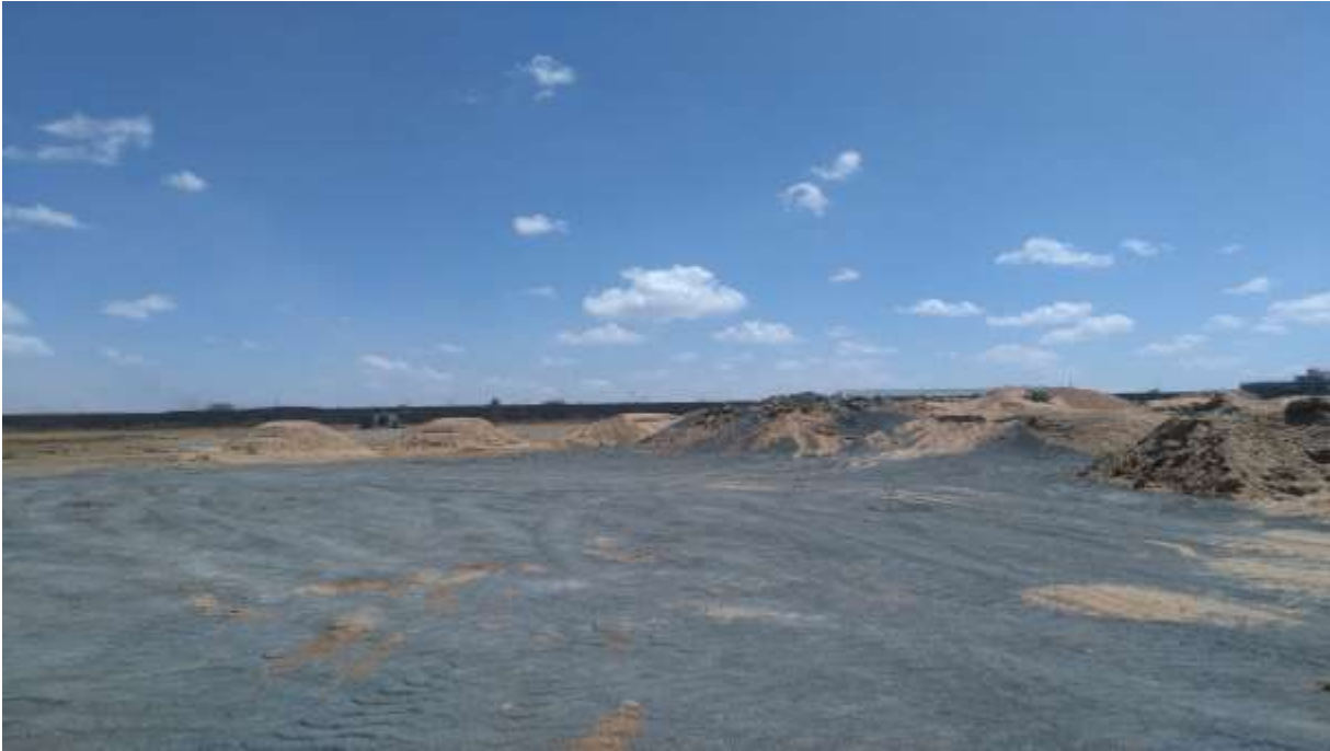
Part of the project site
