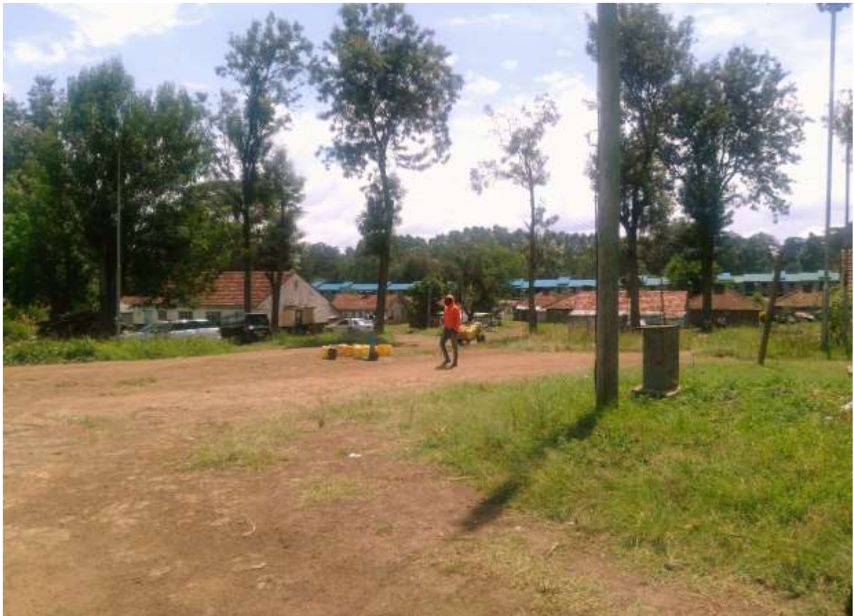
Buildings at the project site to be demolished
