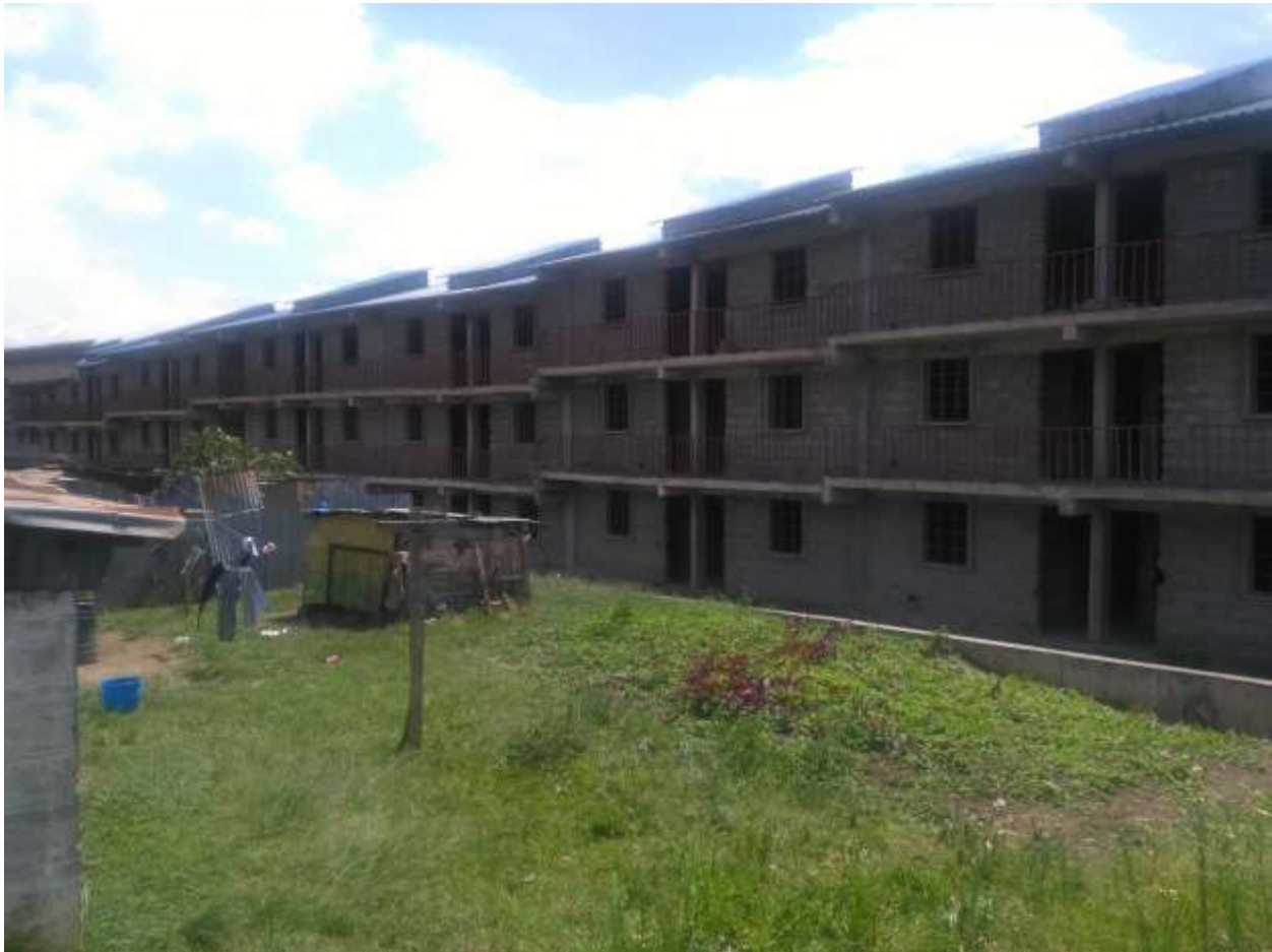
Kenya Railways Staff Houses under construction.
