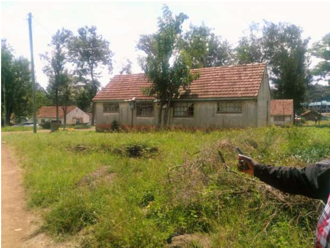
Part of the project site
