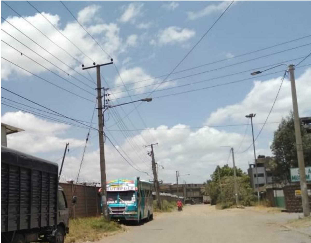
Plate 3.3: Power lines and security lights along Muslim Road
