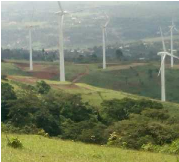
Photo showing Kengen Wind panes
