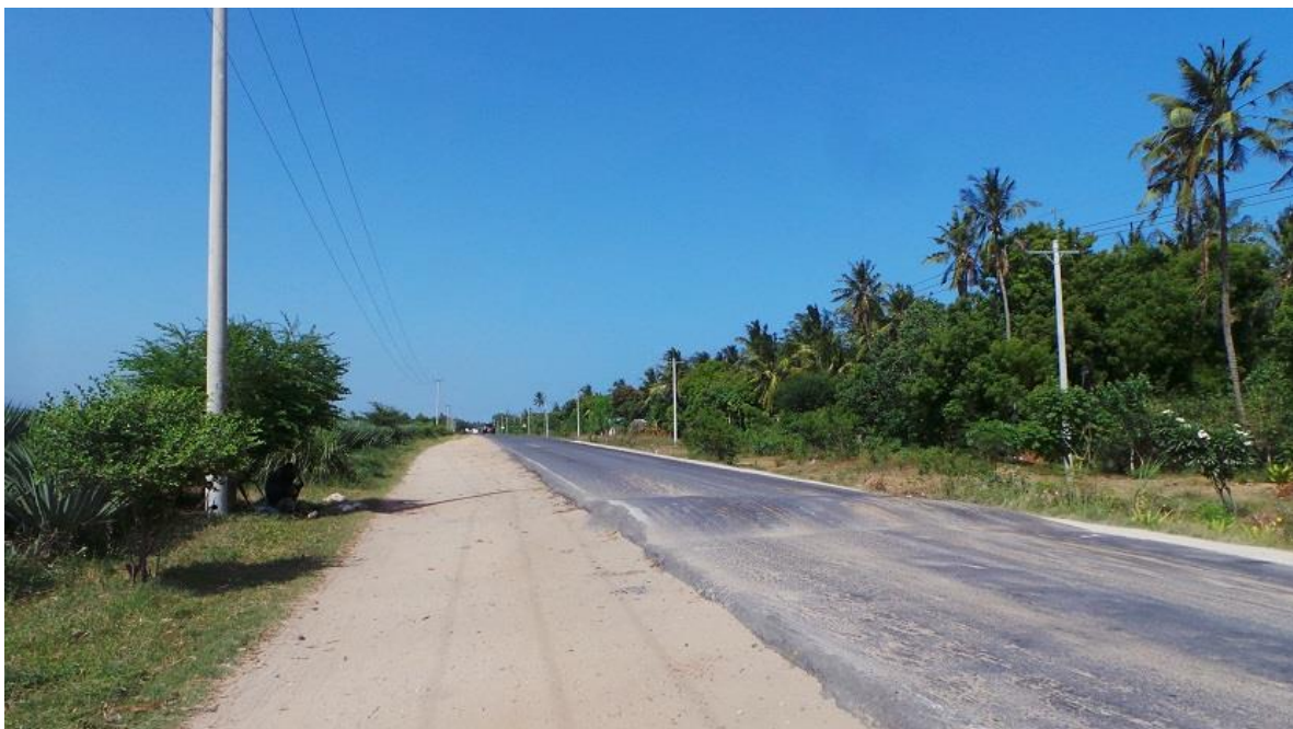
Plate 11: Mombasa-Malindi Highway (B8) passing adjacent the proposed site
