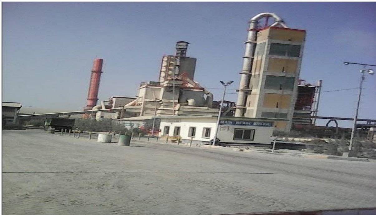
Plate 16: Mombasa Cement Limited in Vipingo area
