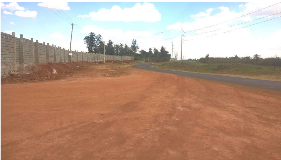
Fig 2.2; the proposed location where a perimeter wall fence is under construction
