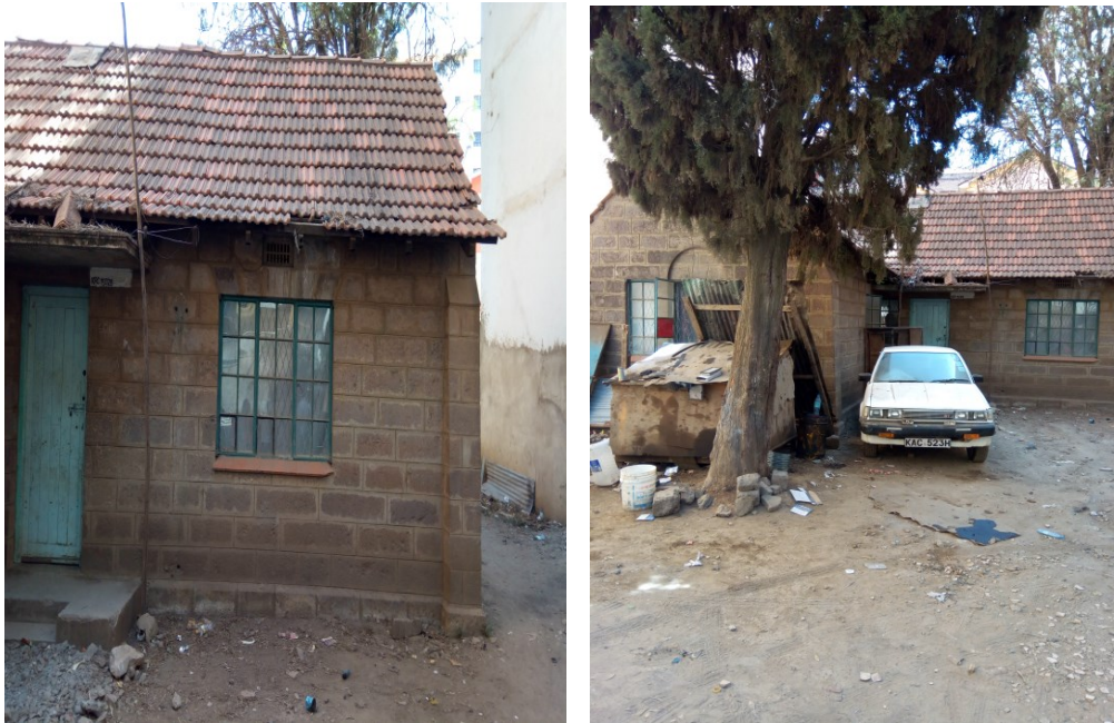
Plate 2: house to be demolished
