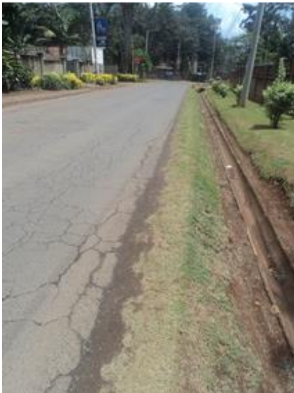
Plate 4: Access Road to site (Riverside Drive)
