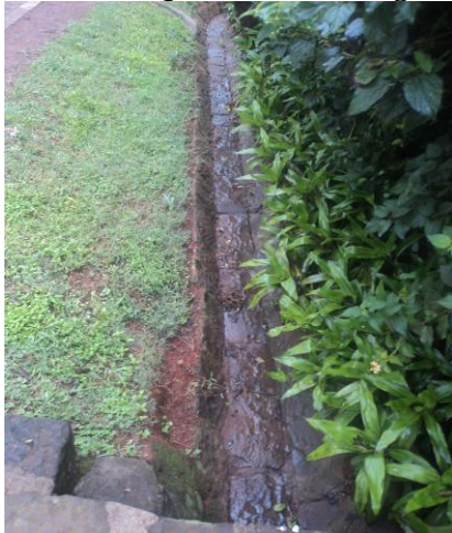
Plate 10: Open drains along the road
