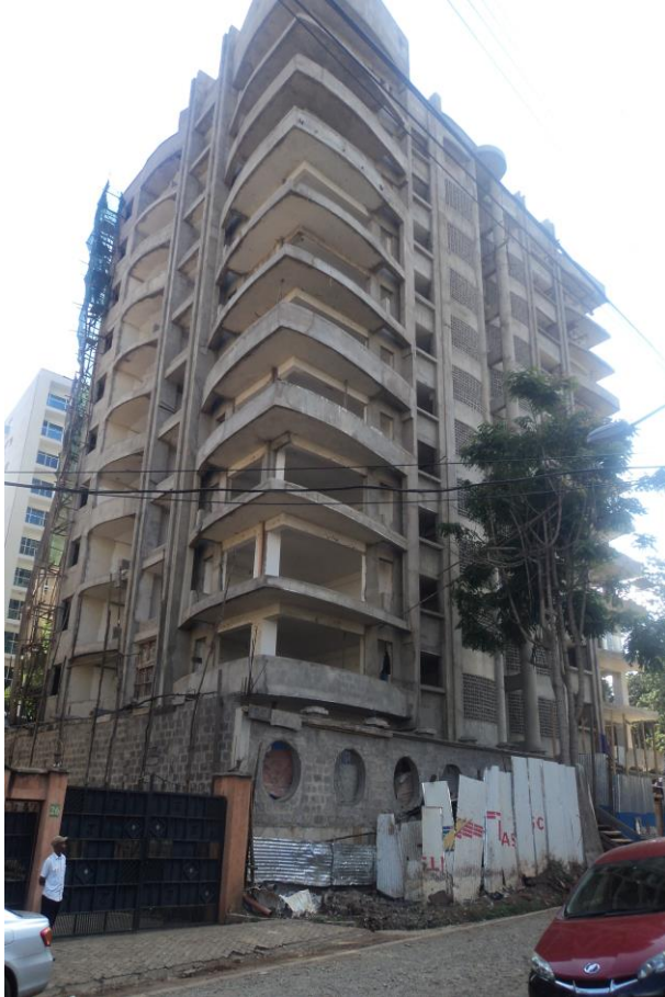
Plate 1: Ongoing Construction of Westin Apartments
