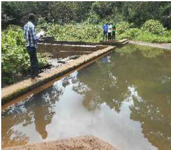
Intake Works on Tungu River for Kiang'onde Treatment Works
