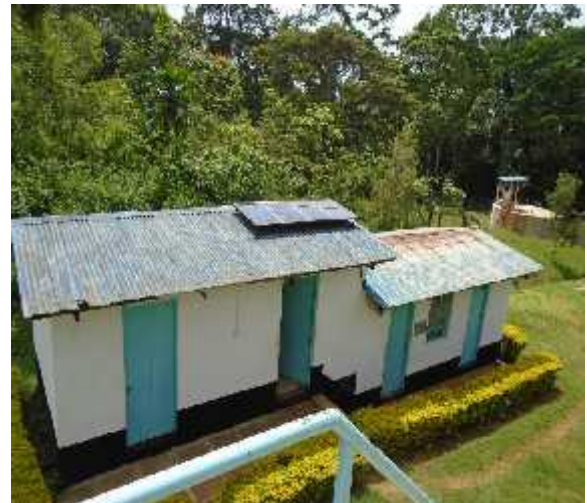
Operator's Office, Laboratory and Chlorine Store at Kiang'onde Treatment Works.
