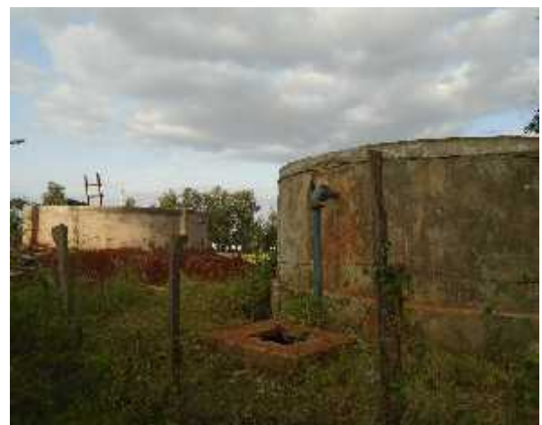
Existing NIWASCO 100m 3 capacity Storage Tank adjacent to a local Community Scheme & 100m 3 capacity Storage Tank at Makawani School
