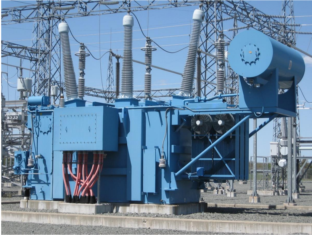
Figure 4: Power transformer image courtesy of MGB Electrique
