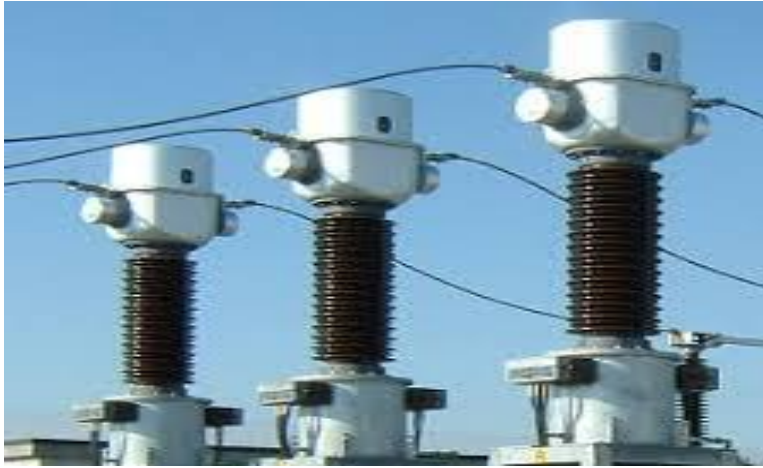
Figure 6: Image of current transformers
