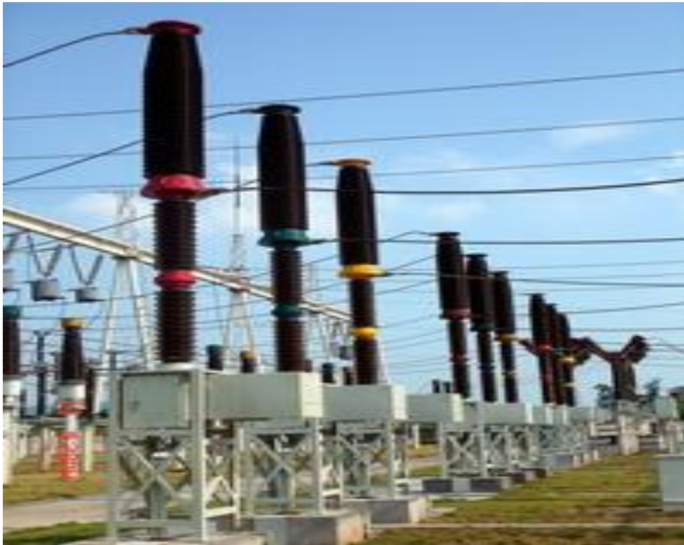
Figure 5: Circuit breaker Image of a single pole circuit
