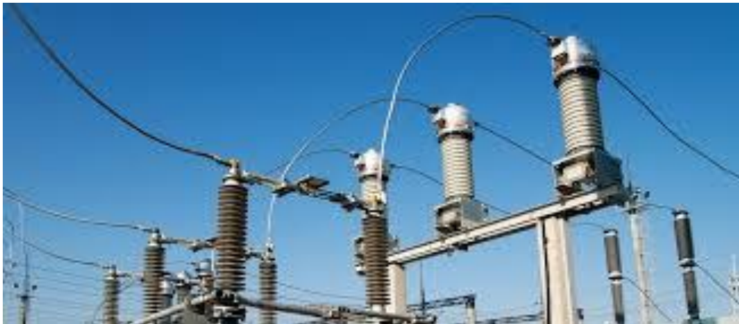
Figure 7: Capacitor Voltage Transformers With and Without Wave Trap. Courtesy of KPLC
